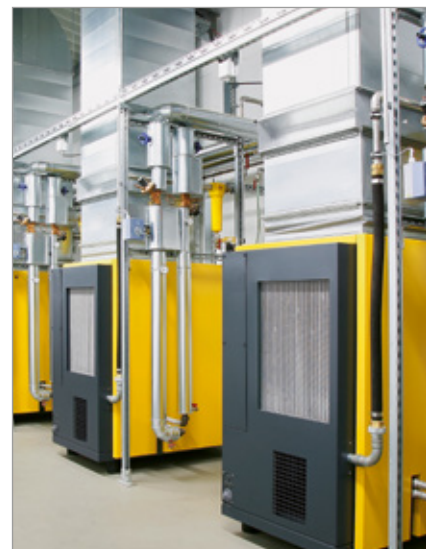
Fig. 2: Correct connection of compressors to a heat recovery system
