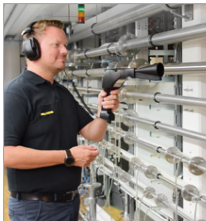
Fig. 4: Locating leakages using ultrasound
