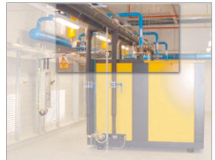
Fig. 3b: Vibration-damping compressor connection with axial compensator
